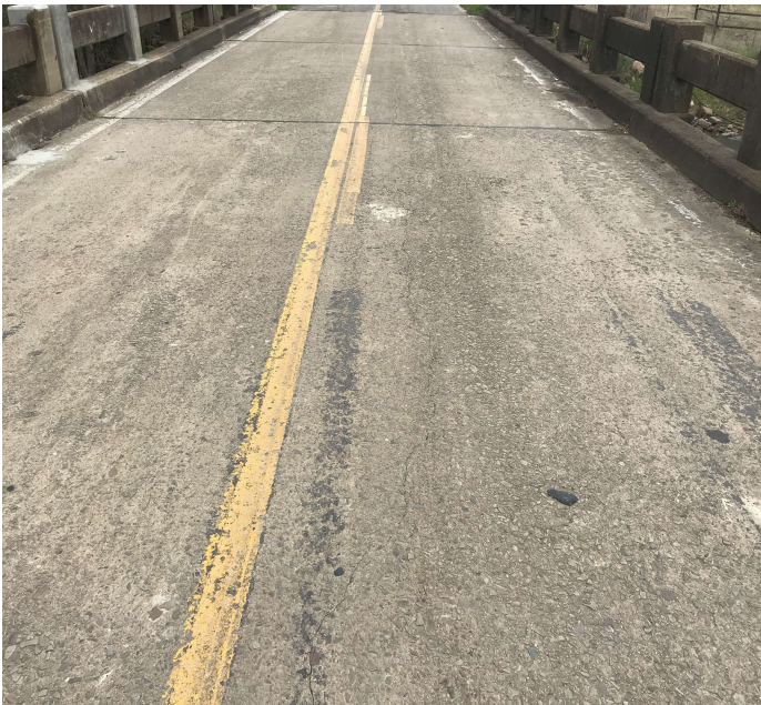
PHOTO 1 Description Sealable deck cracking.
