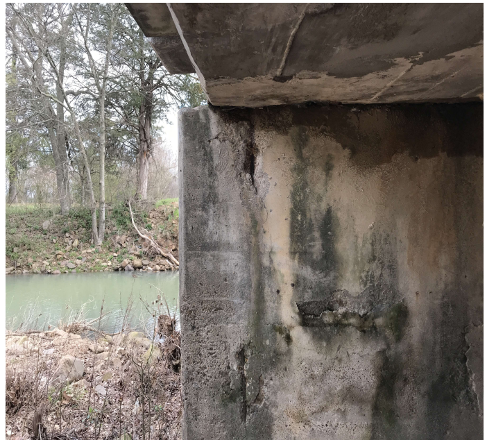
PHOTO 2 Description Bent # 2 Lt spalling with exposed reinforcing steel.
