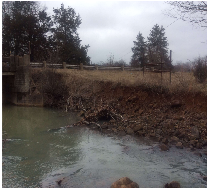
PHOTO 2 Description Some erosion with loss of riprap adjacent to the wingwalls photo of southeast wingwall.
