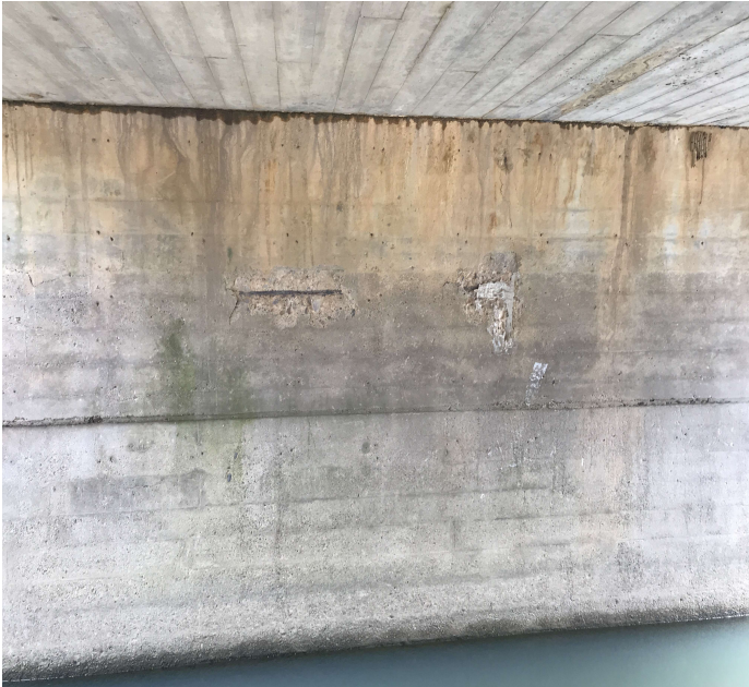
PHOTO 3 Description Bent # 3 Span # 2 spalling with exposed reinforcing steel.
