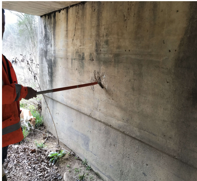
PHOTO 1 Description Bent # 2 Span # 2 spalling with exposed reinforcing steel.
