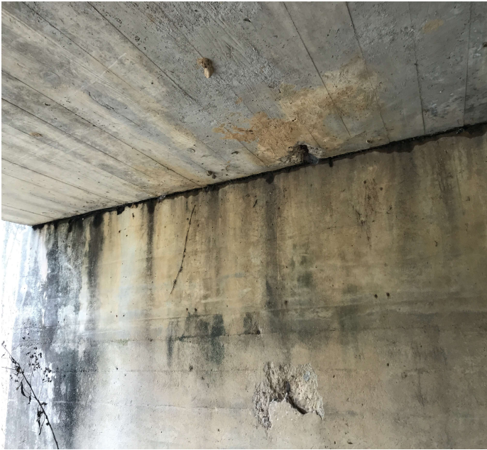
PHOTO 1 Description Span # 2 & 3 shallow spalling with exposed reinforcing steel on the undersurface of the slab.
