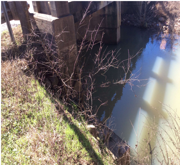
PHOTO 1 Description Minor erosion at Bent 4, wing walls. Bent 4 Lt pictured.
