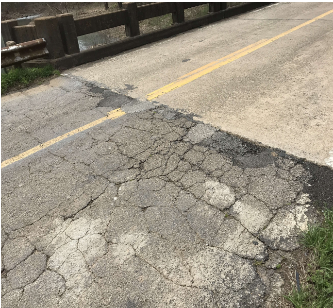
PHOTO 1 Description Asphalt settlement and deterioration at the east approach.
