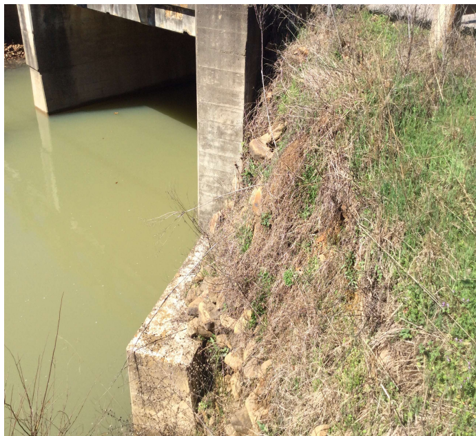
PHOTO 3 Description Minor erosion at Bent 4, wing walls. Bent 4 Rt pictured.
